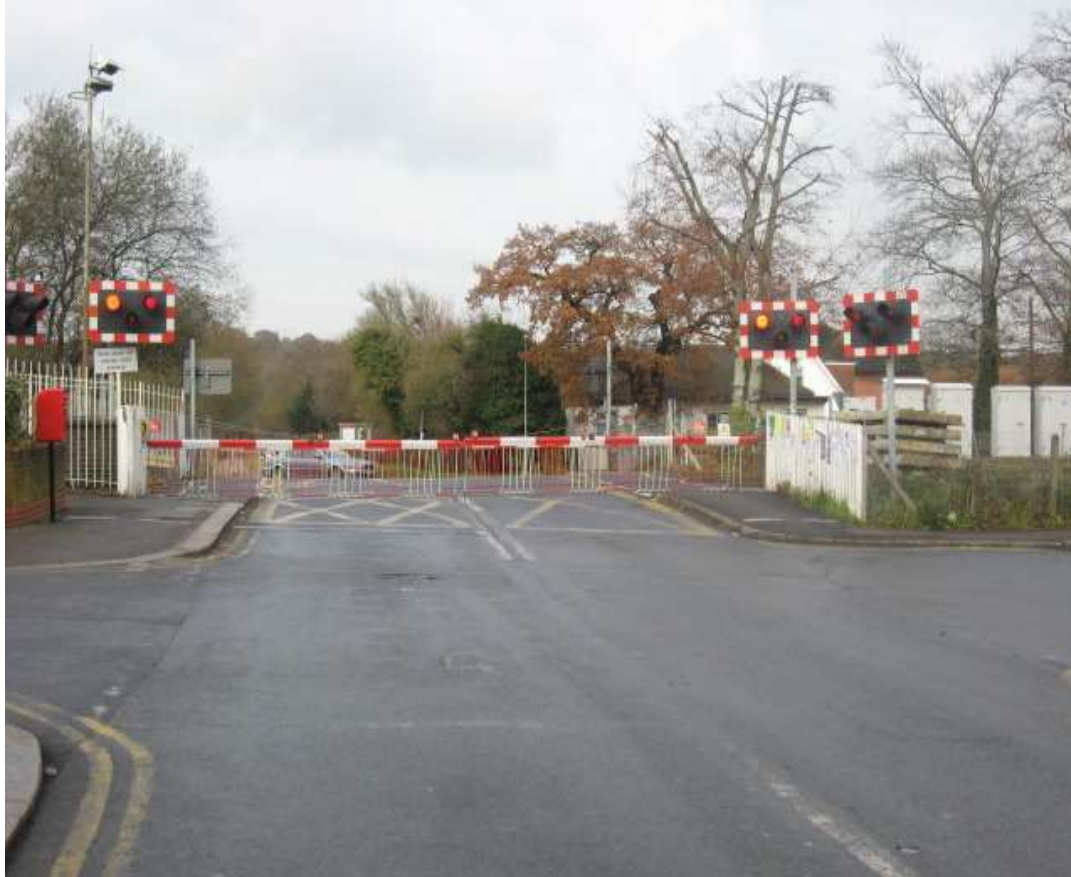
Ashtead MCB CCTV
